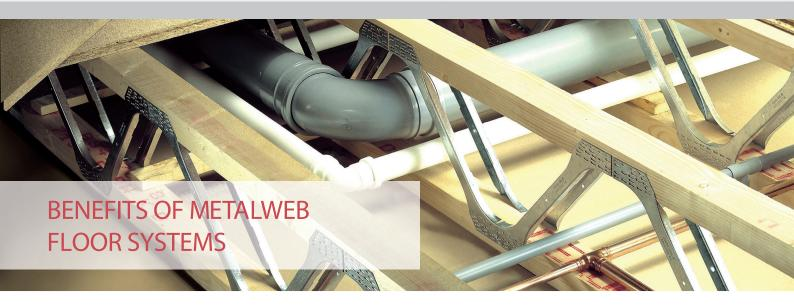
Constructed of kiln dried stress graded timber and plated together with high strength steel webs, metalweb floor systems have a number of benefits compared with other floor and joist systems.
