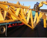
The FLT Operator shall reverse slowly, lowering the boom of the truck as they move back. NEVER stand in the area around the lorry or where the lorry will move into, or allow any others to enter the danger area.
