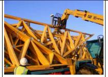
NEVER stand between the forklift and the trailer, or under or on the forks, or allow any others to enter the danger area.
