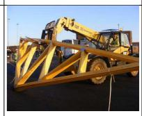
When the truss is at its lowest, the FLT Operator shall reverse back, removing their forks from the truss. The apex is supported by the tyre.
