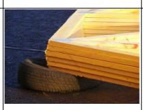
The FLT Operator shall re-position his vehicle and slide the forks in where they can lift the truss and pick them up. The FLT Operator shall then move them to the compound.
