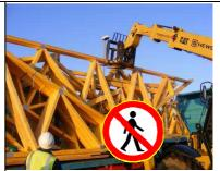
The Driver shall release the individual band / rope attaching the bundle to the lorry. This should be completed from the ground using the telescopic cutters provided. The driver must be in a safe position when carrying out this function
