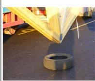
The apex of the truss to be placed in the tyre.
